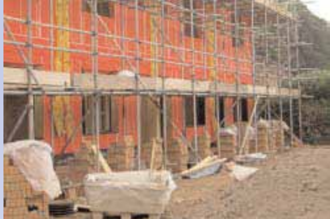
Linx Homes: Park Avenue, Louth under construction
