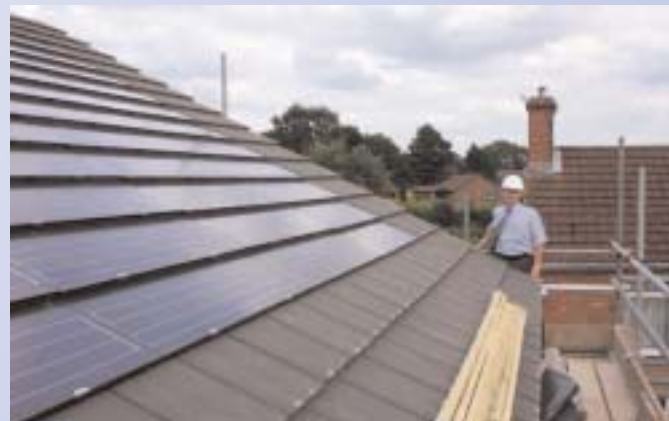
Photovoltaic roof cells: Franklin Gardens, Spilsby
