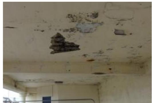
GL 1-2, BB-AA Mt Joint cracks, rust, spalling & hollow Conc. Half cell survey
