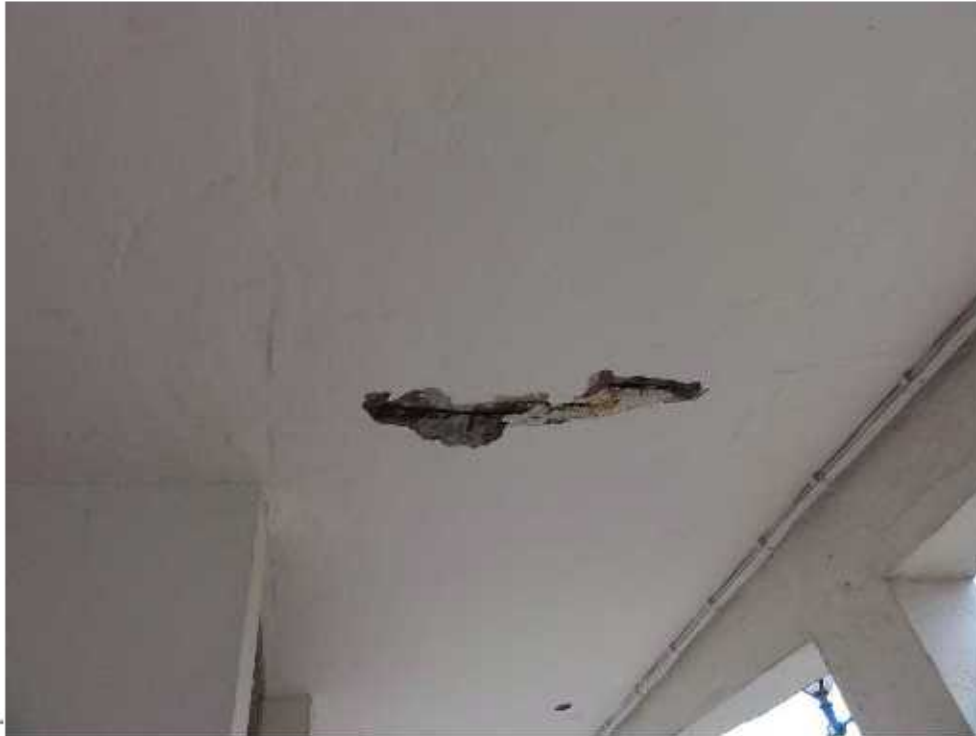
Photo no 11. Soffit of slab at crack GL D, 1-2, concrete crack and spalling.
