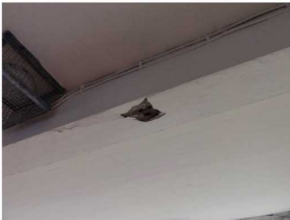
Photo no 6. Cross beam GL 2 C-D concrete spalling.
