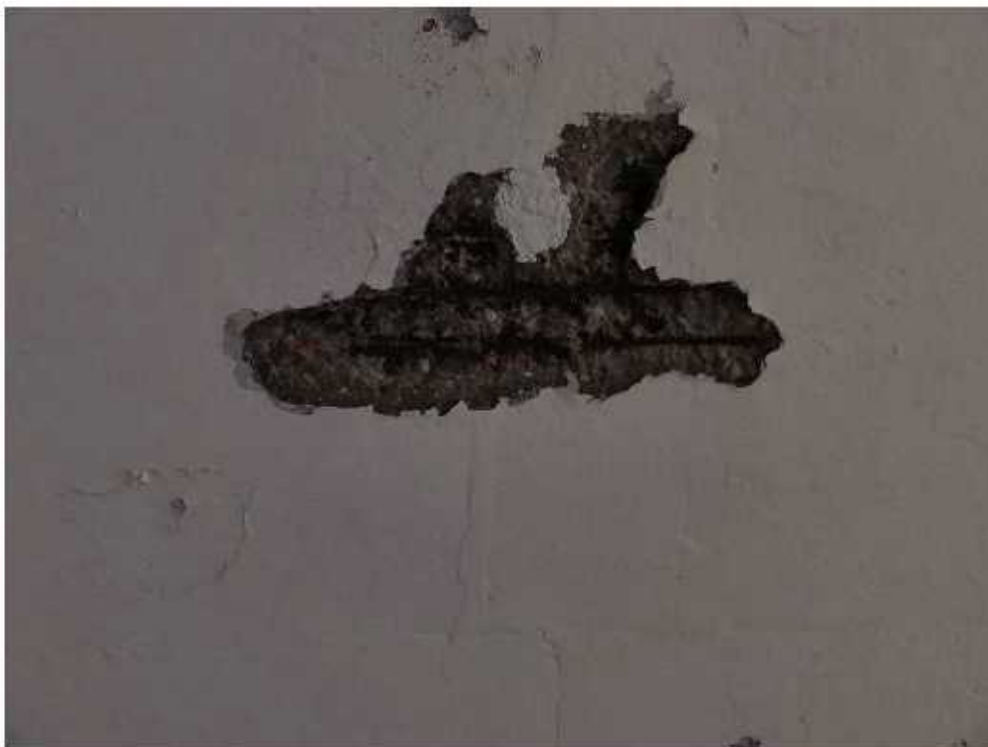
Photo no 10. Soffit of slab GL 1-2, C-D hollow concrete & spalling.
