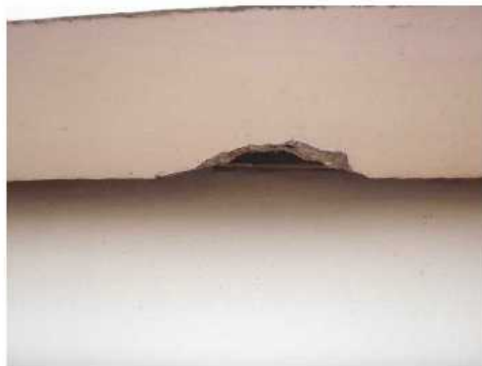
Photo no 4. Fascia beam GL 1, F-G (near café) concrete spalling.
