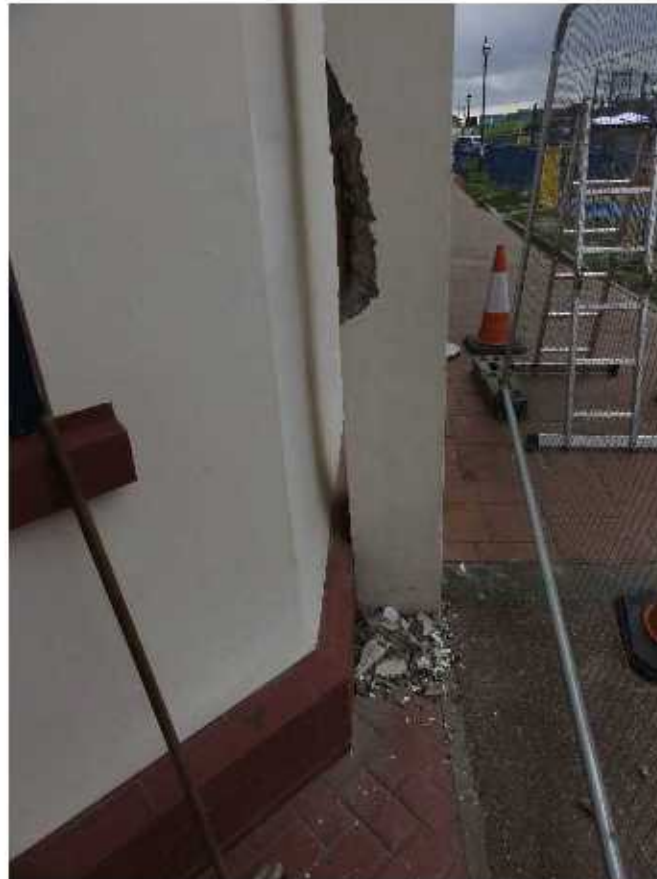
Photo no 3. Column 1E Spalling.
