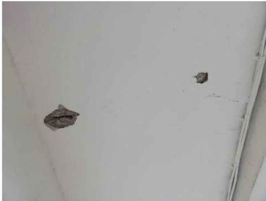
Photo no 9. Soffit of slab GL 1-2, C-D hollow concrete & spalling.
