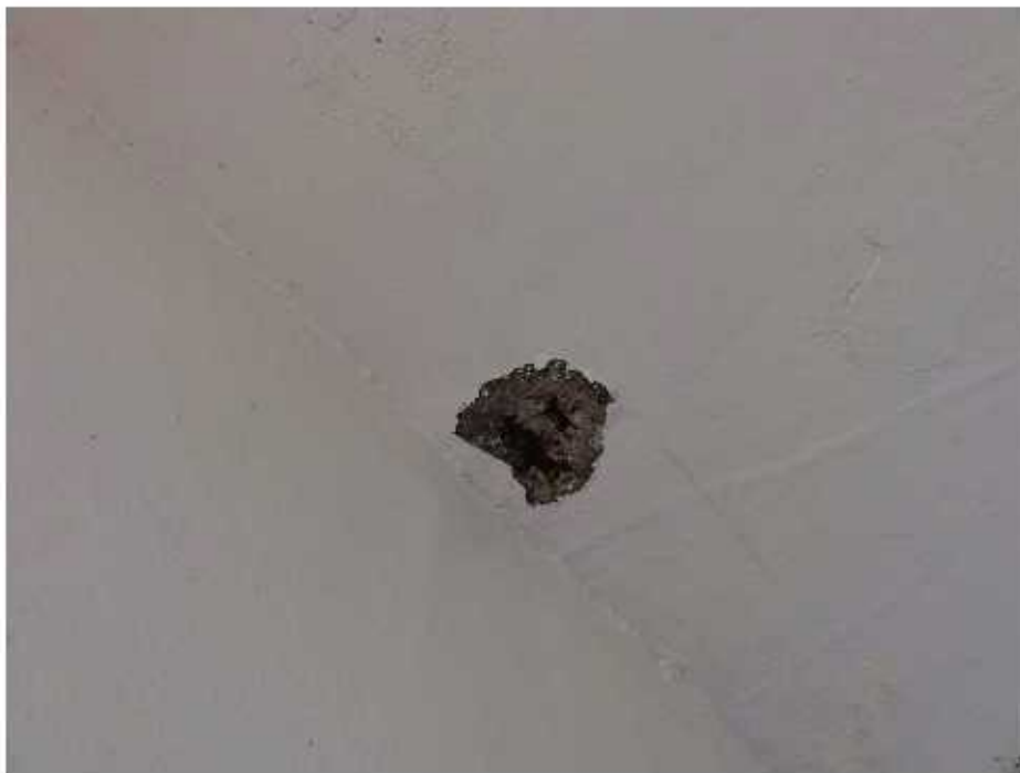
Photo no 8. Soffit of slab GL C, 1-2, hollow concrete & spalling.
