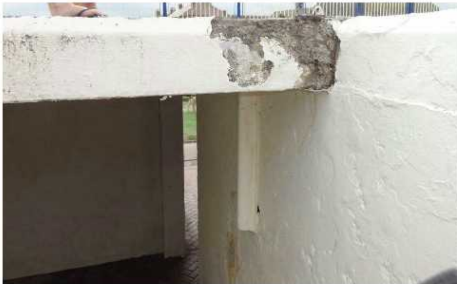
Photo no 7. Edge of slab over North staircase, concrete spalling near balustrade anchor bolt installation.
