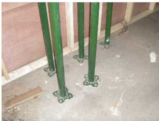
Photo no 2. Temporary props at GL 1H structural joint, secured to floor.
