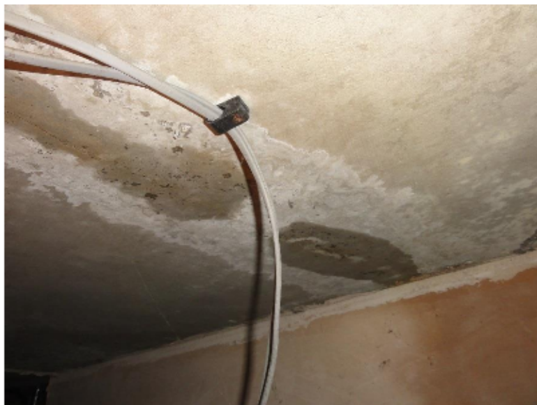
Photo no 19. Crack through roof slab above Café with damp patches at GL 1-2, E-F.
