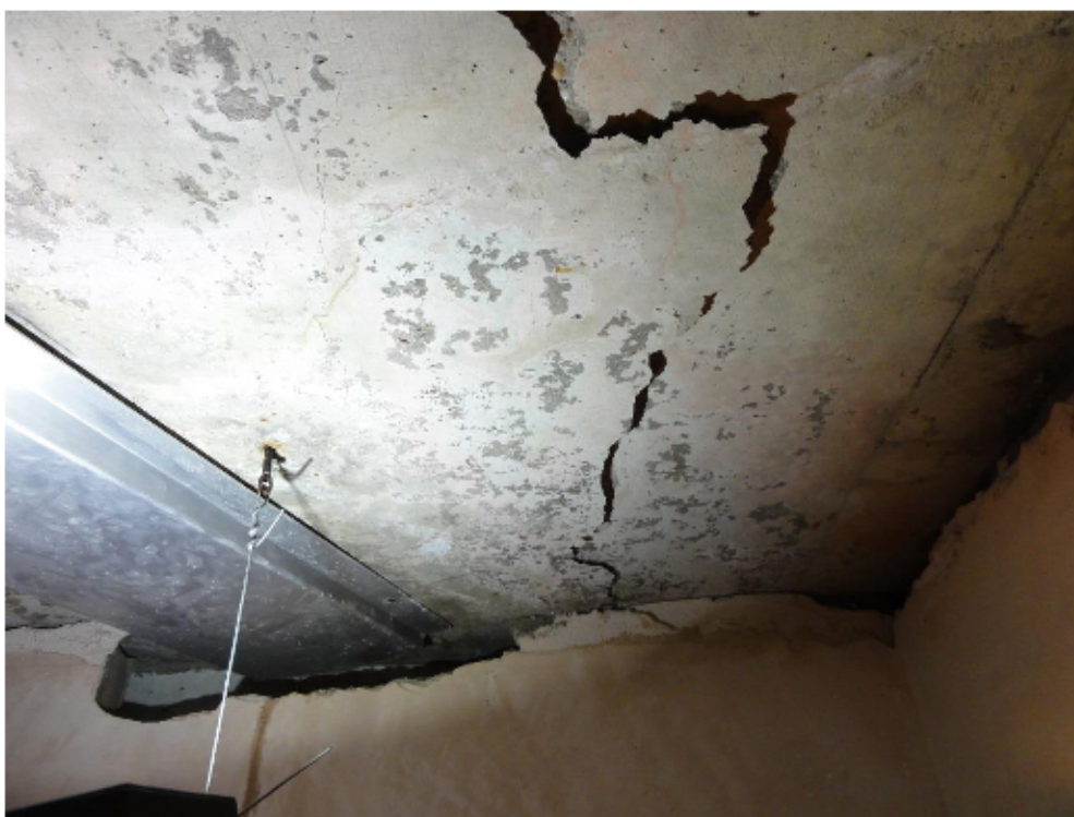
Photo no 22. Crack through roof slab above Café internal toilet, with steel drip tray (approx. GL 1-2, D-E.)
