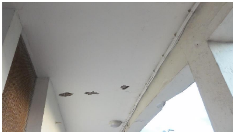
Photo no 14. Soffit of slab GLs 1-2, D-E, further shallow spalling on a hairline crack. Reinforcement corroded with a small loss of cross sectional area.
