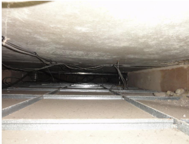
Photo no 5. Slab soffit above suspended ceiling in Cafe showing spalled concrete to the RHS.
