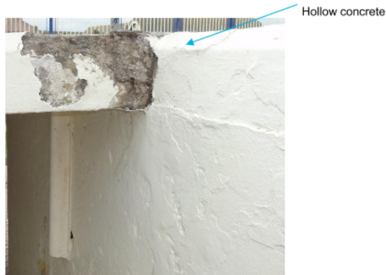
Photo no 13. Top of stair wall alongside north staircase (GL 3, C-D), hollow concrete detected adjacent to RHS of concrete spalling.
