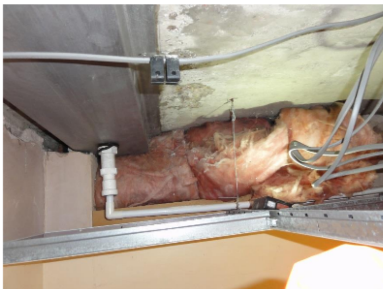
Photo no 21. Crack through roof slab above Café freezer with steel drip tray at GL 1-2, D-E.
