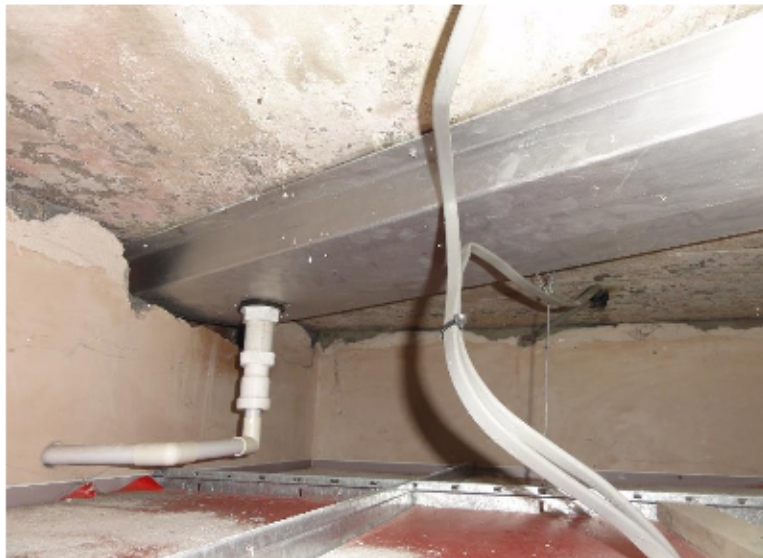
Photo no 23. Spalling and a dripping water leak in ceiling void of Café at GL 2, E-F
