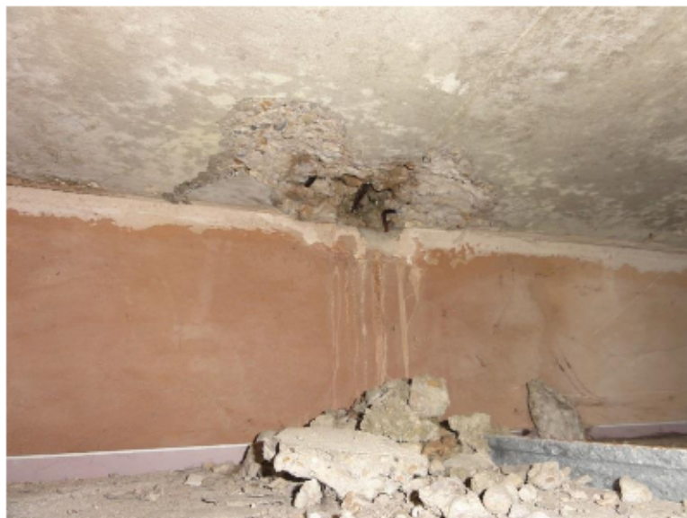
Photo no 24. Spalling and a dripping water leak in ceiling void of Café at GL 2, E-F above internal block wall and under chalet no 2.
