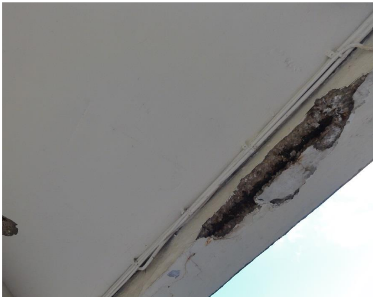
Photo no 9. Further spalled concrete cover from down-stand arched soffit fascia beam GL 1, D-E.
