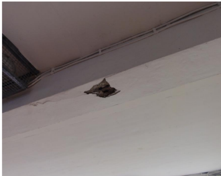
Photo no 12. Cross beam GL 2 C-D further concrete spalling. Reinforcement corroded with only a slight loss of cross section.
