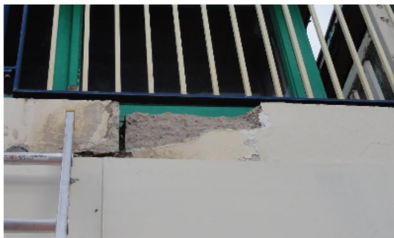
Photo no 7. Half-lap joint on fascia beam GL 1, G-H, showing area of further spalling on RHS
