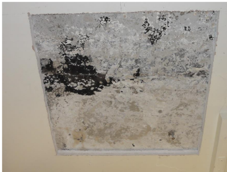
Photo no 18. Exposure in plasterboard ceiling to ice-cream kiosk showing hairline crack in slab soffit at GLs 1-2, B-C with some minor spalling. Black staining damage reported to be from an earlier fire.
