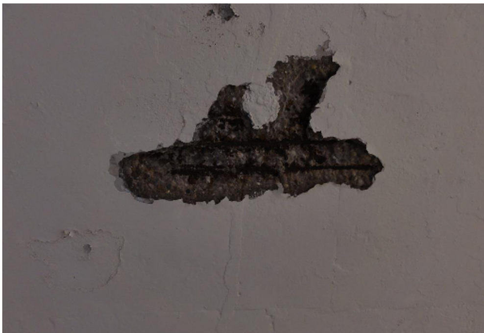
Photo no 16. Soffit of slab at GLs 1-2, C-D showing spalled concrete, corroded reinforcement with loss of cross section.
