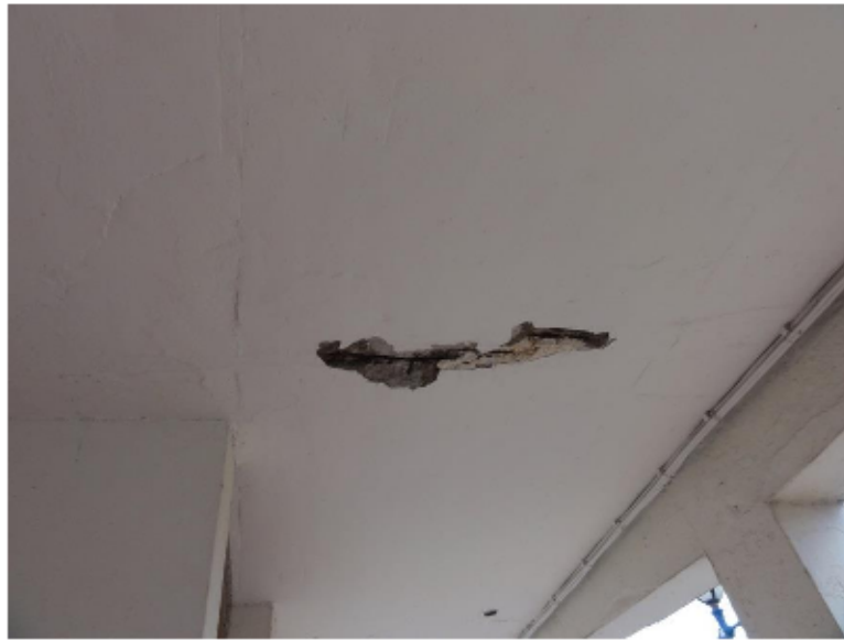
Photo no 15. Soffit of slab at crack GLs D, 1-2, concrete crack and spalling.
