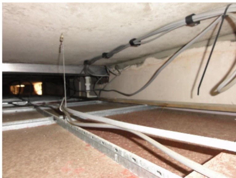
Photo no 6. Slab soffit above suspended ceiling in Cafe showing services & steel drip trays fixed under leaking cracks through roof slab.
