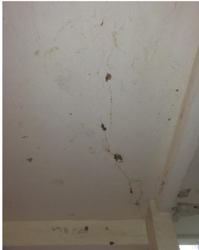
Photo no 17. Hairline crack in slab soffit at GLs 1-2, C-D with some minor rust stains and spalling.
