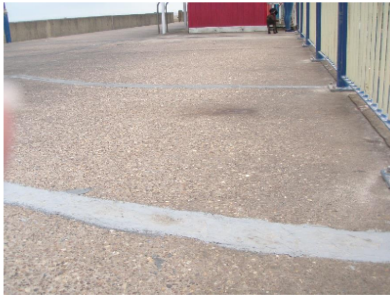
Photo no 25. Repaired cracks in slab at promenade level which approximately correspond with cracks in Garden Café ceiling below. (GL 1-2-3, D-F).
