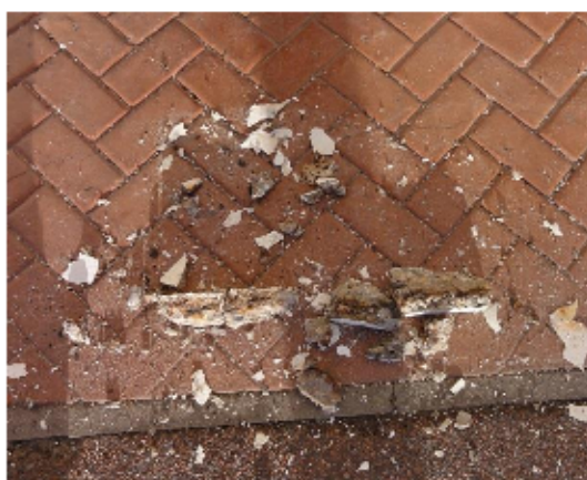
Photo no 10. Close up of spalled concrete from down-stand arched soffit fascia beam GL 1, D-E
