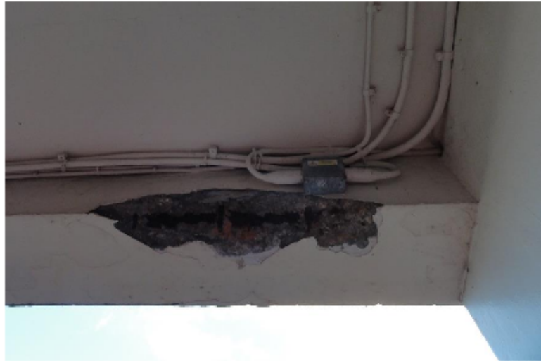
Photo no 11. Small increase in concrete spalling area to edge of down-stand fascia beam at GL 1, C-D near Ice-cream kiosk.
