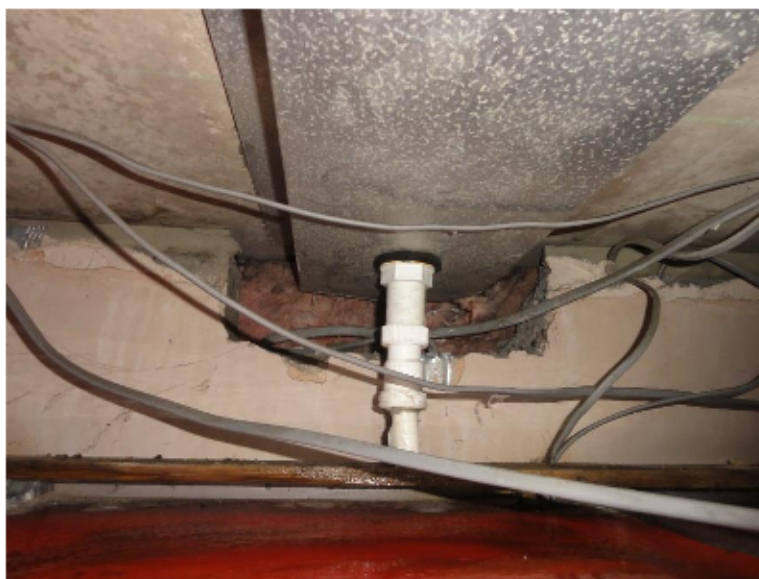
Photo no 20. Crack through roof slab above Café with steel drip tray at GL 1-2, E-F. Drain pipe from drip tray leaking water onto ceiling tile above electric deep fat fryer.
