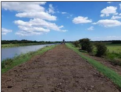
Permanent repairs to the breach were completed at the start of August. The Environment Agency (EA) put 50 steel piles weighing 40 tonnes (the same as five HGVs) into the embankment where the breach took place. Clay and stone were placed either side of the piles to cover and re-instate the embankment. Top soil has been placed ready for grass-seeding in
