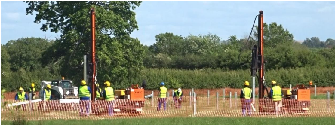
Insert 3: Machinery Installing Solar PV Framework Legs
