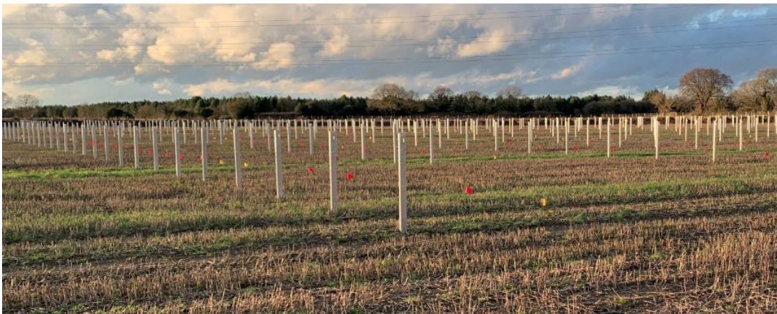
Insert 4: Photograph Following Installation of Legs
