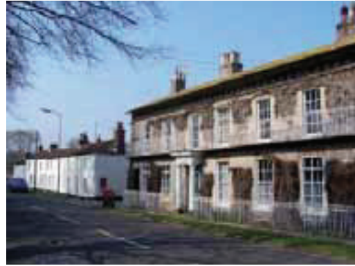
Salem House & Nos. 1-9 Station Road
