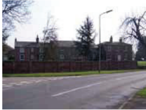
The Grange, Boston Road
