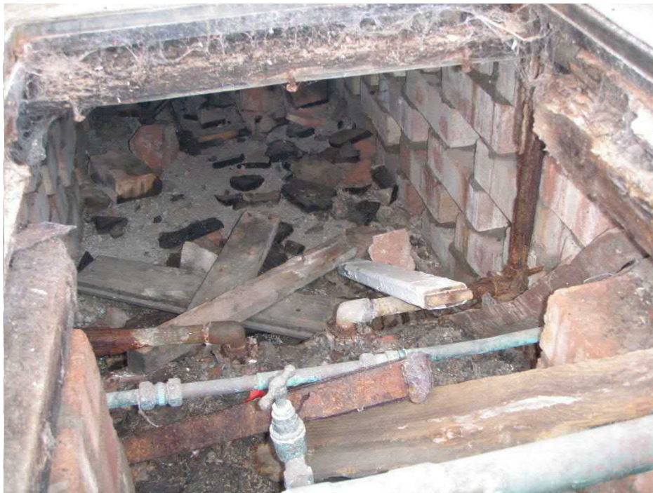
Photo no 21: Under croft to huts nos 23-24 in central section showing water and drainage services.
