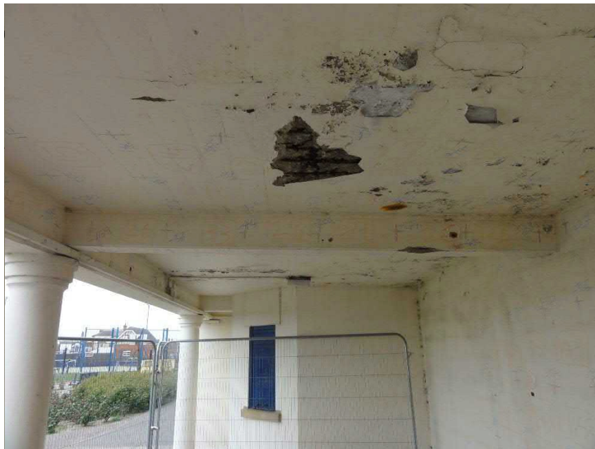
Photo no 11: Slab soffit rust stains, cracks and spalled concrete GL 1-2, U-V.
