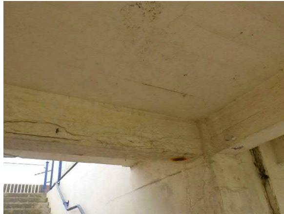
Photo no 24: Cross beam over central stair access GL 2 Z-AA showing rust staining, cracking and hollow concrete.
