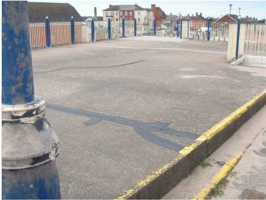
Photo no 08: Floor slab at promenade level GL B-D, 1-3 North end showing shrinkage cracks and mastic asphalt remedials to kiosk roof in distance.
