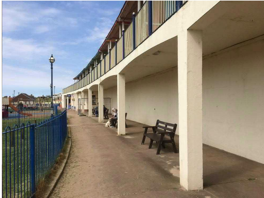
Photo no 04: Colonnade to Northern section showing curved profile to fascia beams.
