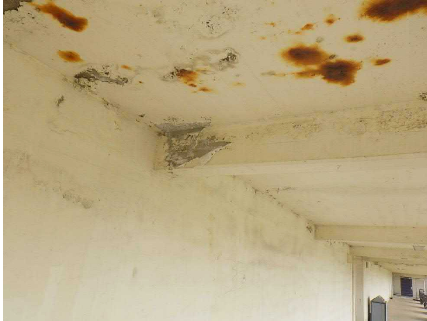
Photo no 14: Slab soffit GL 1-2, CC-MM showing cracks, spalling and rust staining.
