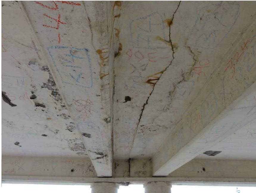
Photo no 12: Down stand transverse beams and movement joint GL 1-2, AA-BB showing spalled and hollow concrete, along with NDT testing chalk notes.
