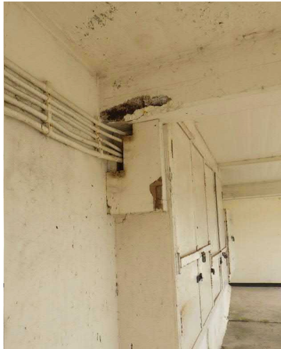
Photo no 09: Cross beam GL P1-2 showing spalled concrete and loss of section to rebar and electrical meter boxes
