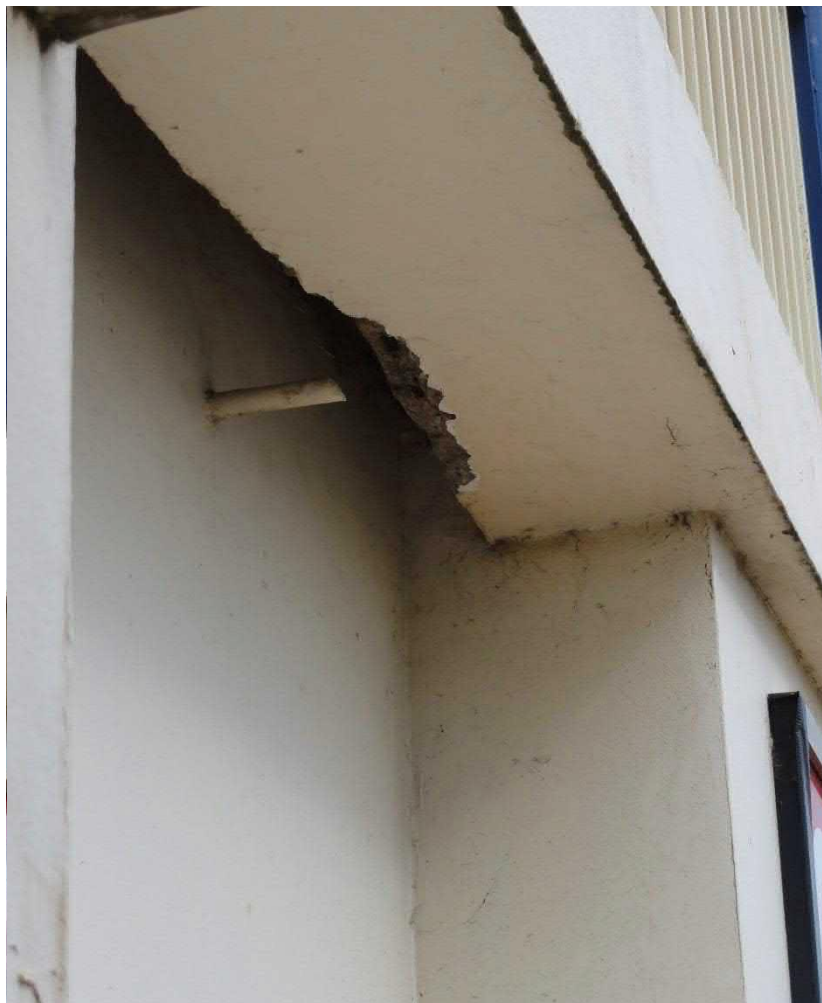
Photo no 03: Showing spalling to fascia beam on GL 1, D near Café.
