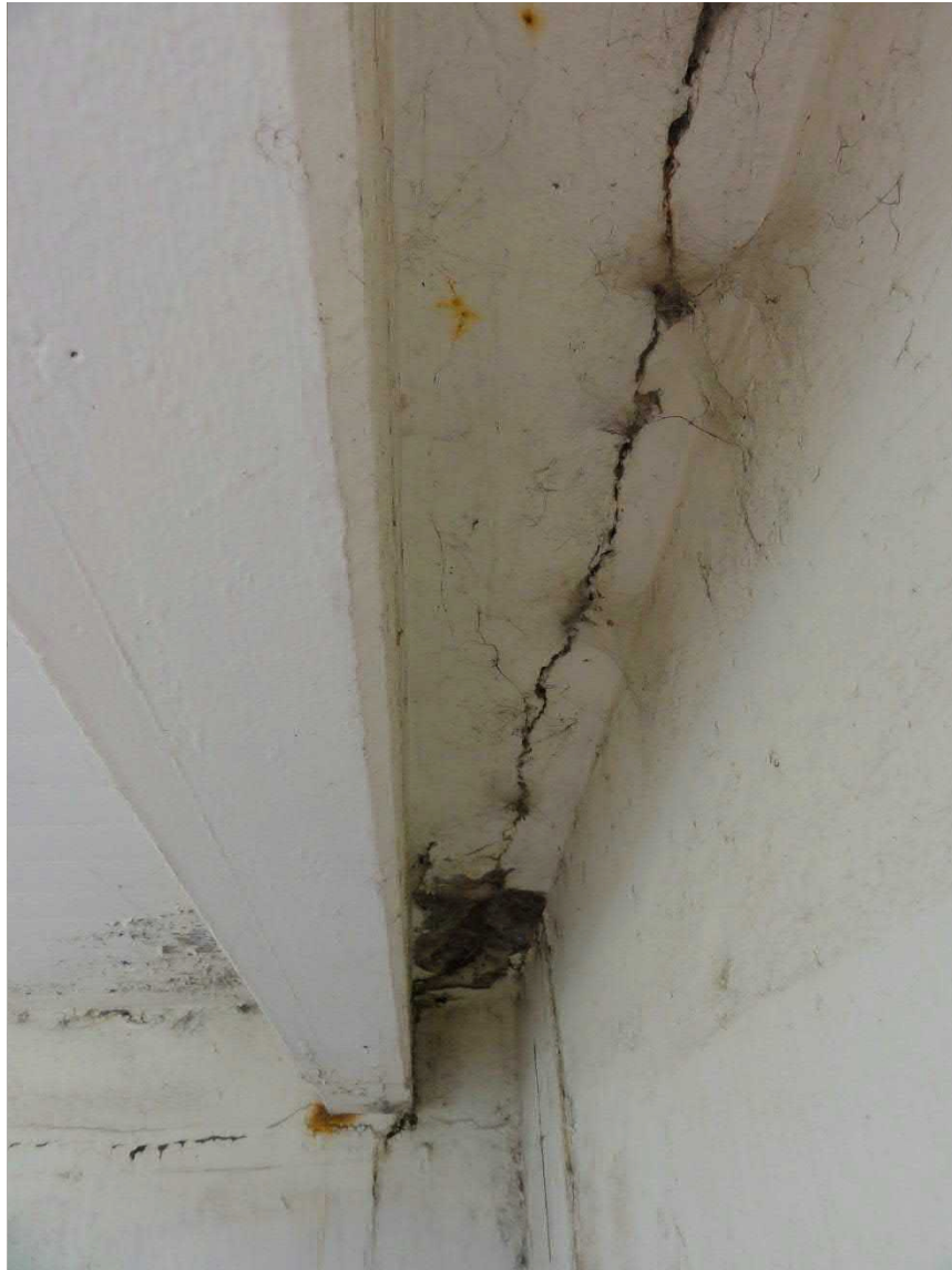
Photo no 16: Movement Joint in slab soffit GL KK, 1-2 showing rust stains and cracking.
