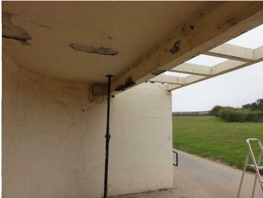
Photo no 17 Cross beams GL 1-2, LL-MM showing severe cracking and spalling necessitating temporary structural support.
