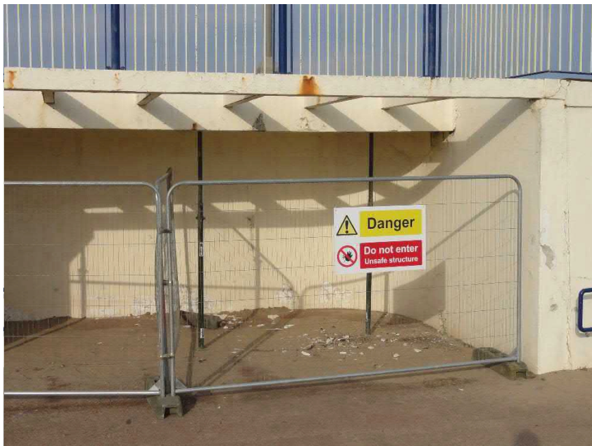
Photo no 18 Cross beams GL 1-2, LL-MM showing severe cracking and spalling and temporary structural support.
