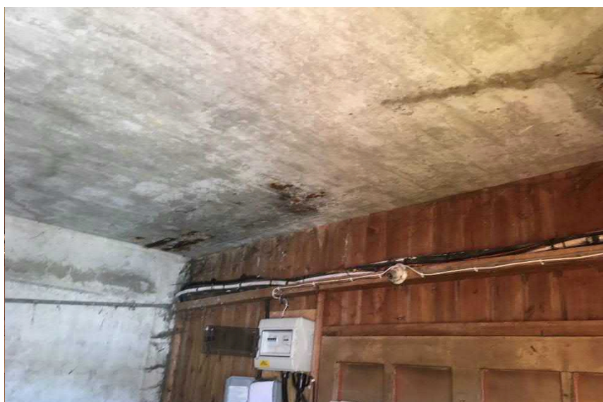
Photo no 10: Slab soffit inside tank room showing spalling, cracks and rust stains. Also a detached electrical services (far wall) [Safety Hazard].
