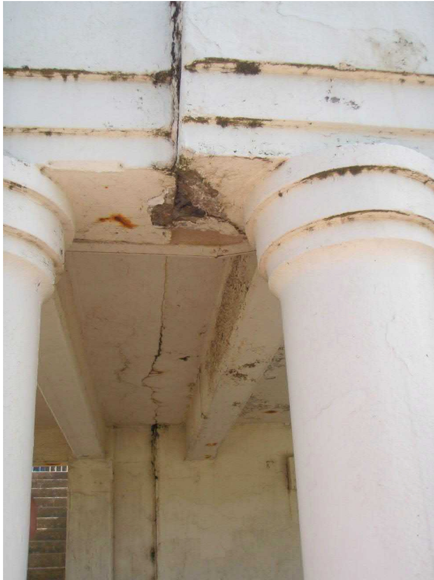
Photo no 15: Spalling at head of column GL 1BB, and exposed aggregate to transverse beam GL BB and movement joint to central stairs
