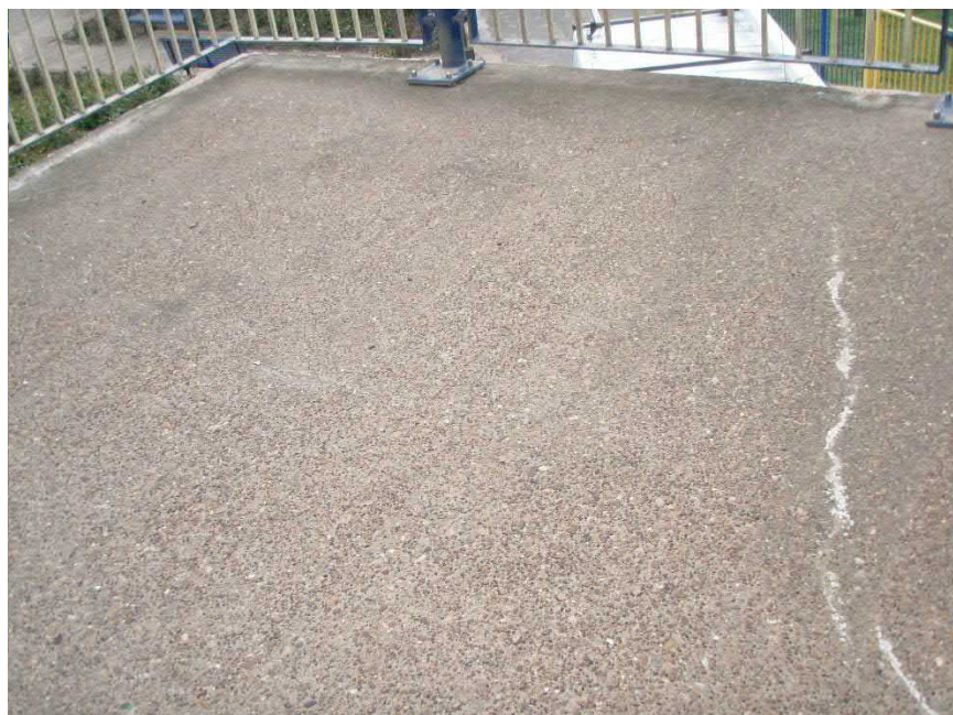
Photo no XX: Slab at promenade level showing shrinkage cracks GL 1-2, M-N.
