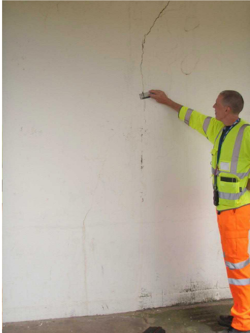
Photo no 07: Shrinkage crack in spine wall near GL N 2.
