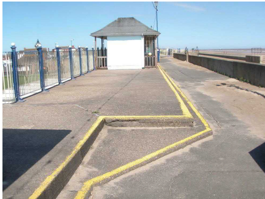
Photo no 20: Promenade slab at GL 2-3, LL-MM showing shrinkage cracks.
