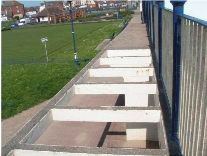
Photo no 19 Small cross beams to fascia beam GL 1, LL-MM showing severe cracking and spalling.
