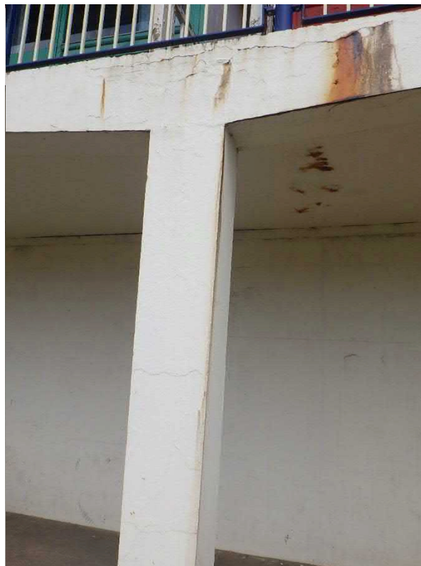
Photo no 23: Fascia beam over column J1 showing rust area and structural crack over column.
