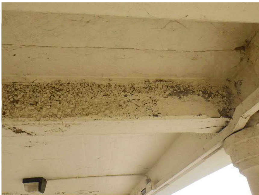
Photo no 13: Transverse beam GL CC, 1-2 with exposed aggregate on side of beam
