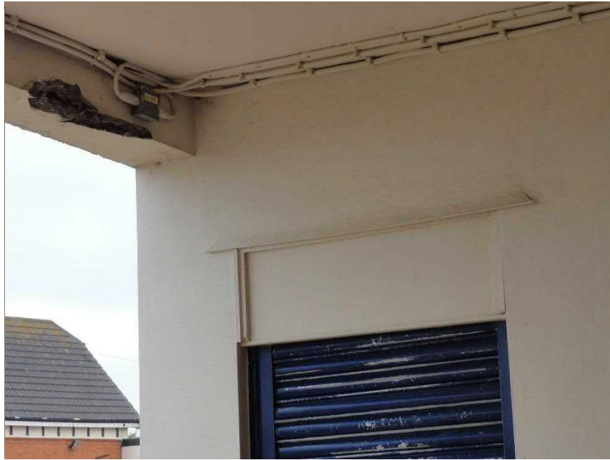
Photo no 02: Showing spalling to fascia beam on GL 1, C-D near Ice Cream Kiosk.
